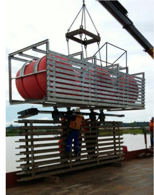
Installation of real size log boom module
